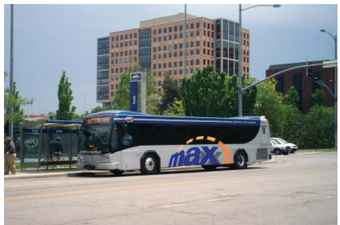
Figure 210.2 Transit stop example. Create and maintain a convenient, pedestrian-friendly environment near stops and stations.
