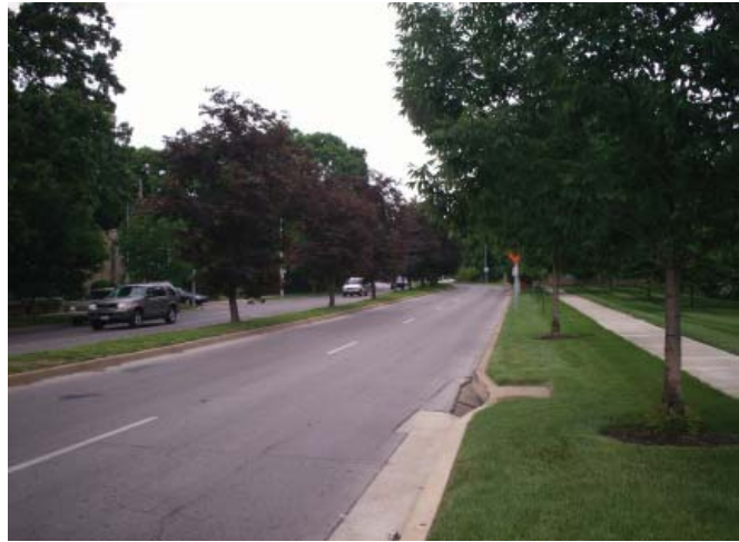
Figure 226.1 Apply medians as part of a corridor access management strategy to improve safety and multi-modal operational efficiency, in situations where traffic volumes and speeds are high.
