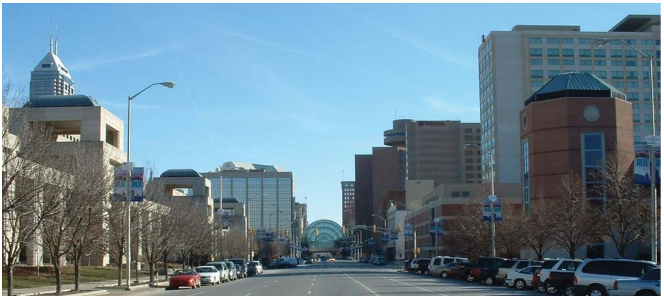
Figure 225.2 Avoid combining minimum widths for vehicle travel way and minimum dimensions on adjacent zones, where it could affect the safety of users by reducing the separations between users.
