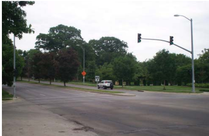
Figure 226.2 Medians in urban areas should only be as wide as necessary to provide the desired function, such as left turns or pedestrian refuge.
